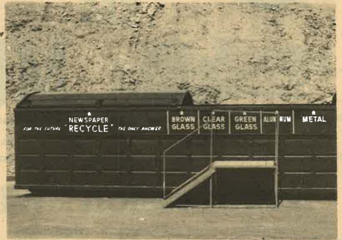
This is the recycling facility at the Red Hill site near Vallecito.
