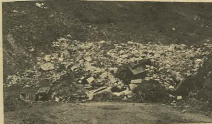
This is the sloped landfill where compacted waste is deposited and covered at the Red Hill site.
