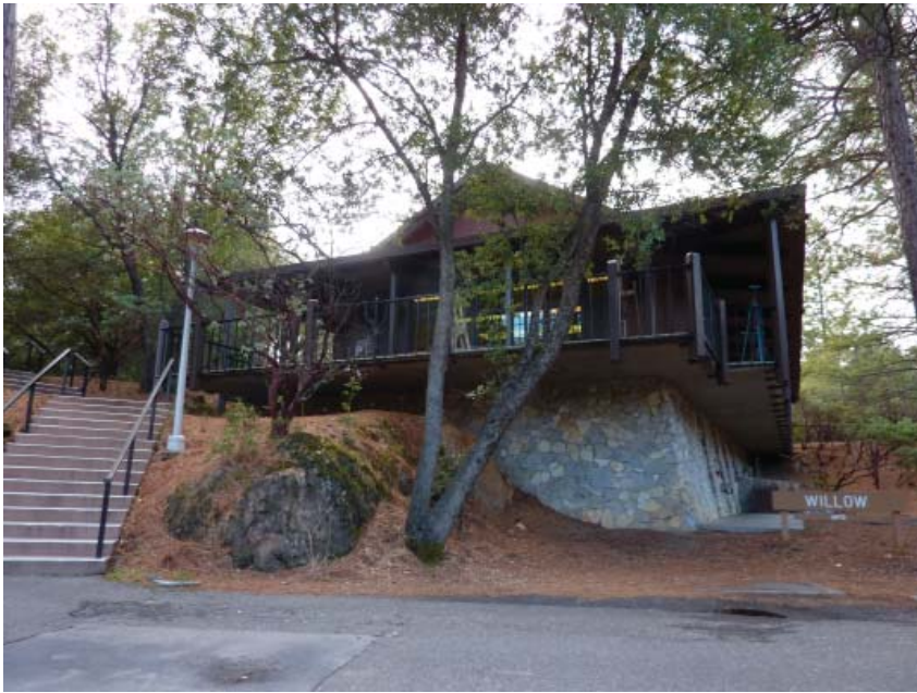
Existing Area near Willow Building
