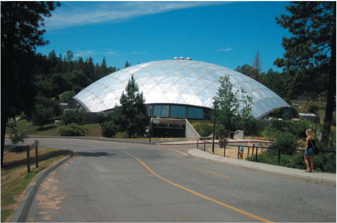
Oak Pavilion - Existing Condition - Before (Image from 2007 Campus Master Plan)
