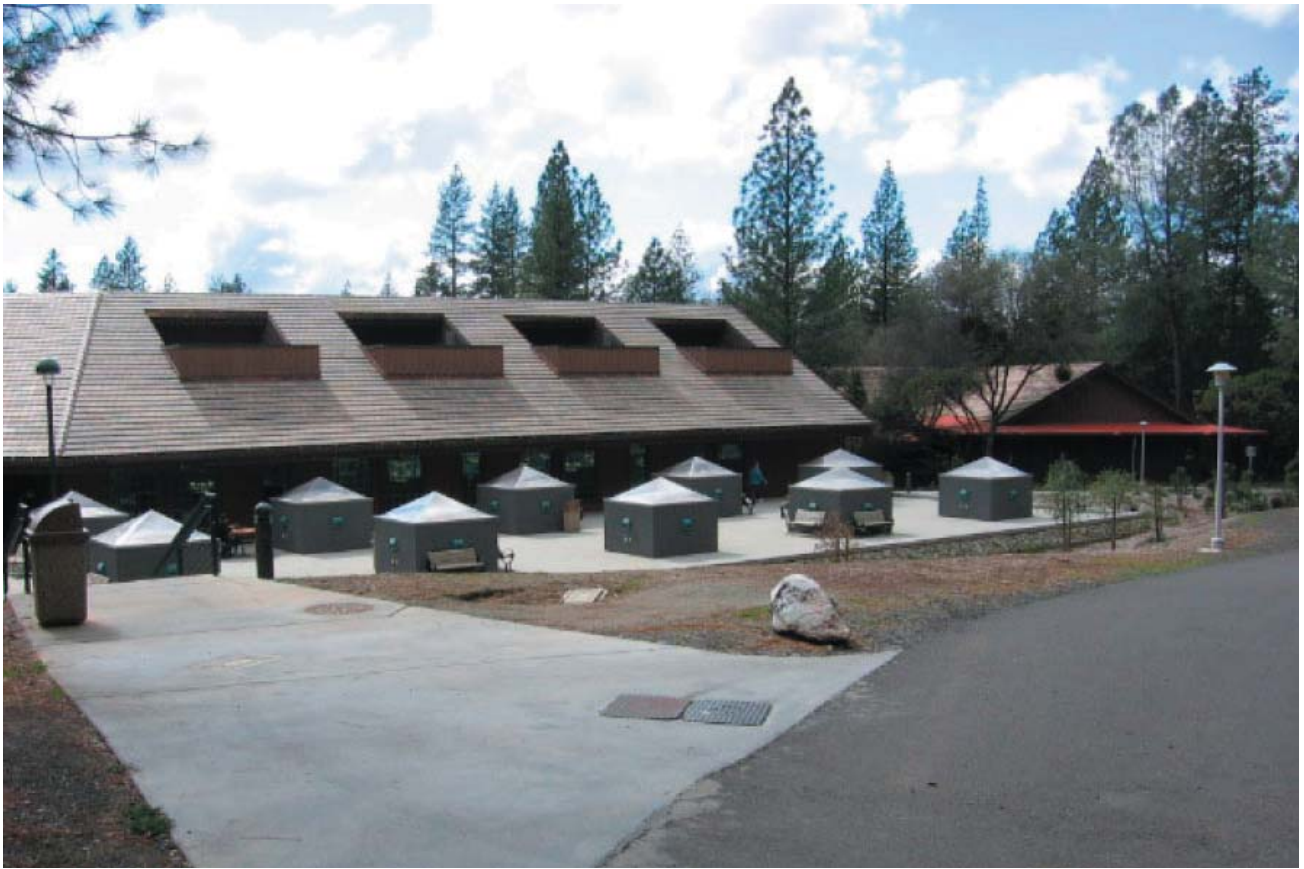
Tamarack Hall - Existing Condition - Before (Image from 2007 Campus Master Plan)
