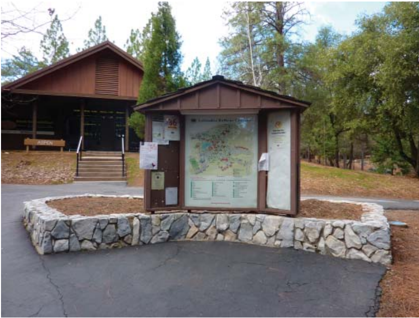
Existing Gathering Area near Aspen Building
